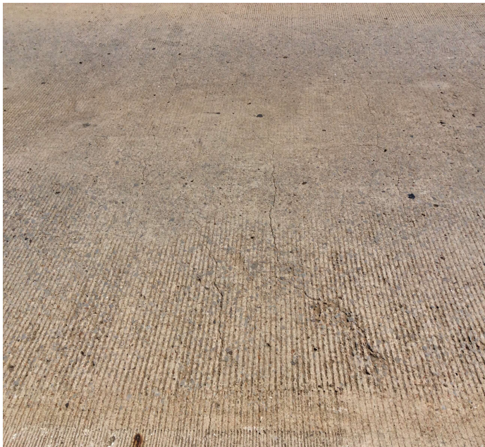
PHOTO 1 Description Span 1. Sealable deck cracks.
