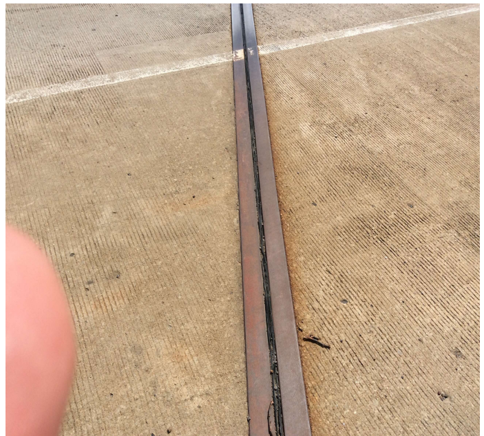
PHOTO 2 Description Span 2 deck joint seal
