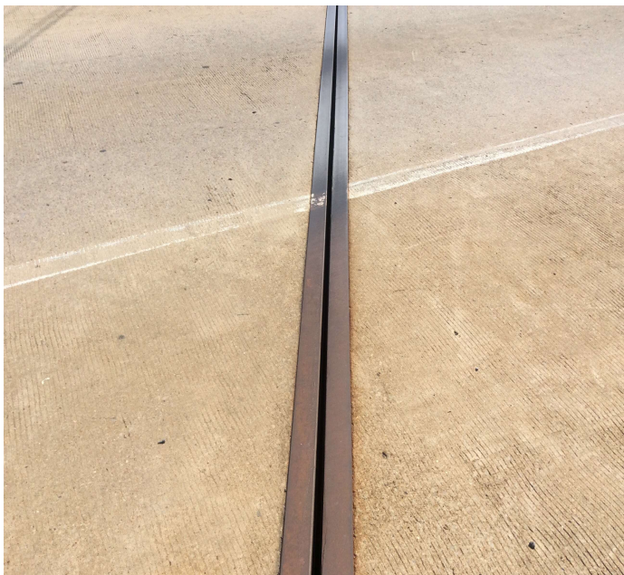
PHOTO 3 Description Bent 4 deck joint seal is missing.
