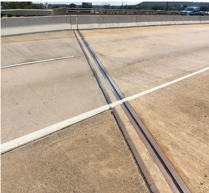
PHOTO 1 Description North abutment expansion joint
