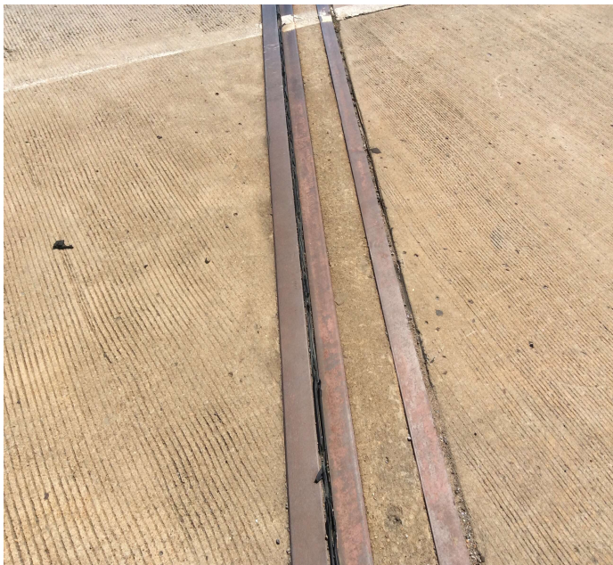
PHOTO 1 Description Span 1 deck joint seal
